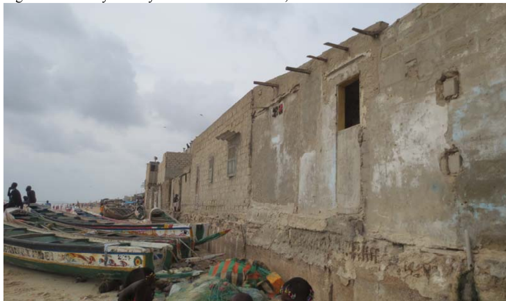
Figure 2: Partially destroyed home in Guet Ndar, Saint-Louis
